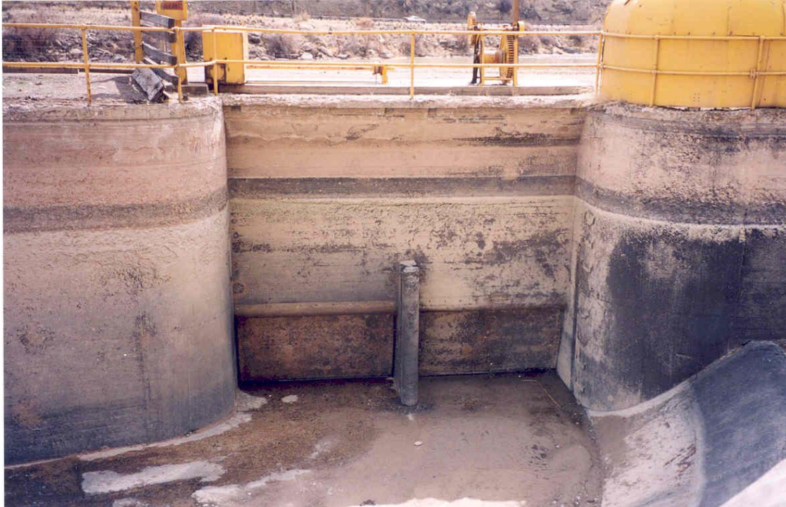
Figure 19. Station 22 spillway. Grand Valley Project RO&M Exam; March 18, 2002.
