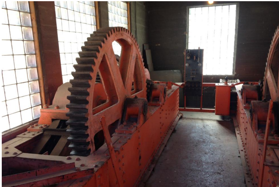
Figure 5. Existing outdated transfer switches and circuit breaker for diversion dam roller gates.
