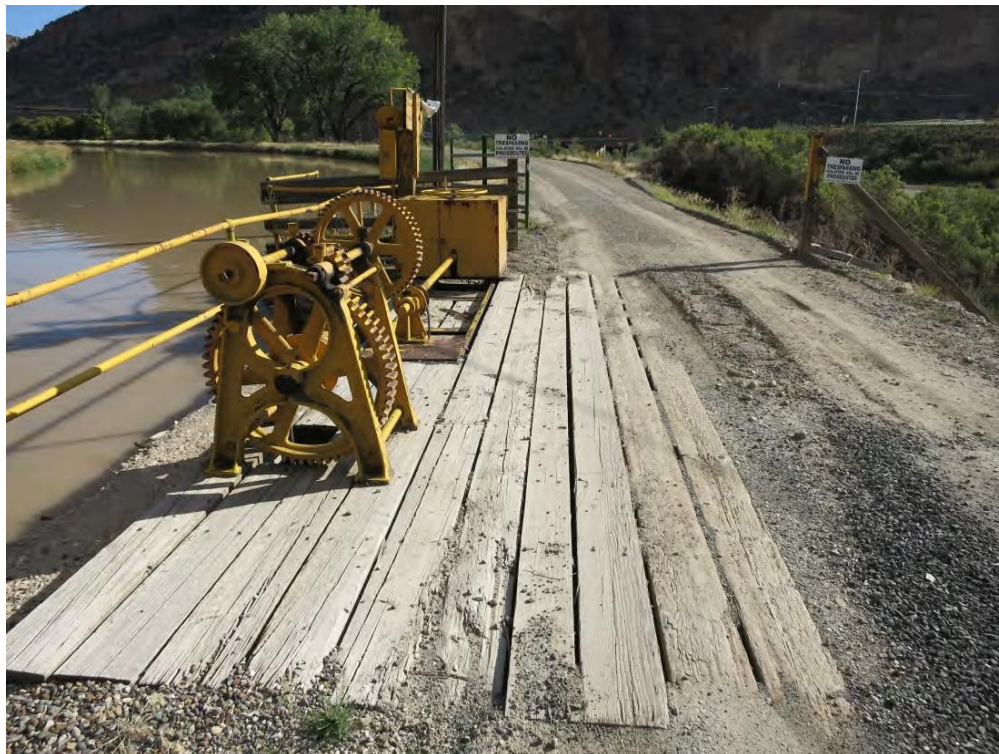
Figure 20. Station 22 spillway. Grand Valley Project RO&M Exam; September 23, 2014.
