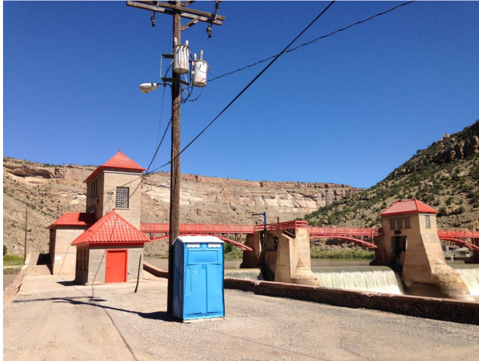
Figure 4. View of existing overhead power lines and the limited space for machinery mobility during mandatory repairs or maintenance on the Dam or canal headworks.
